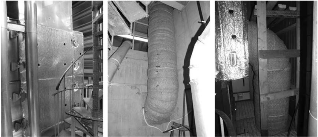
Fig 6. Example of grain dryer insulation.
