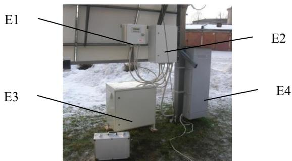
**Figure 4.** Placement of enclosures of electrical equipment: E1 – solar charge controller; E2 – inverter; E3 – VRLA batteries; E4 – dedicated wind turbine charge controller.
