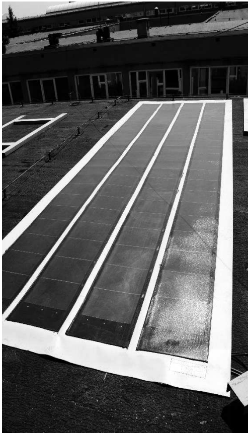
Figure 7. The PV foil with the nominal output peak power 0.406 \text{ kW}_p at the Czech University of Life Sciences Prague.
