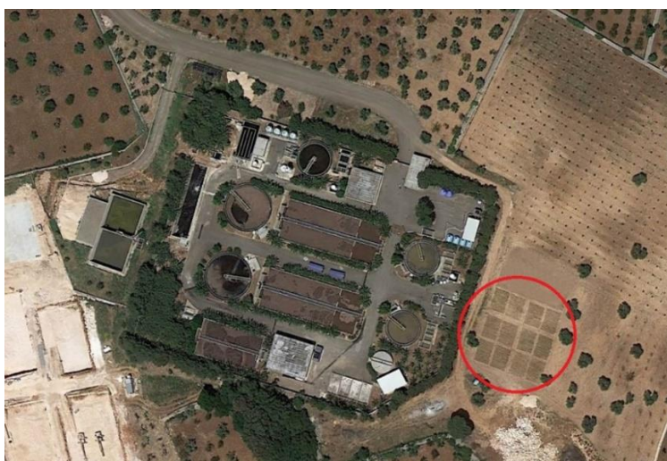
Figure 2. Satellite view of the municipal wastewater treatment plant of Castellana Grotte (Bari, Italy) and experimental field (red circle) ( https://earth.google.com ).
