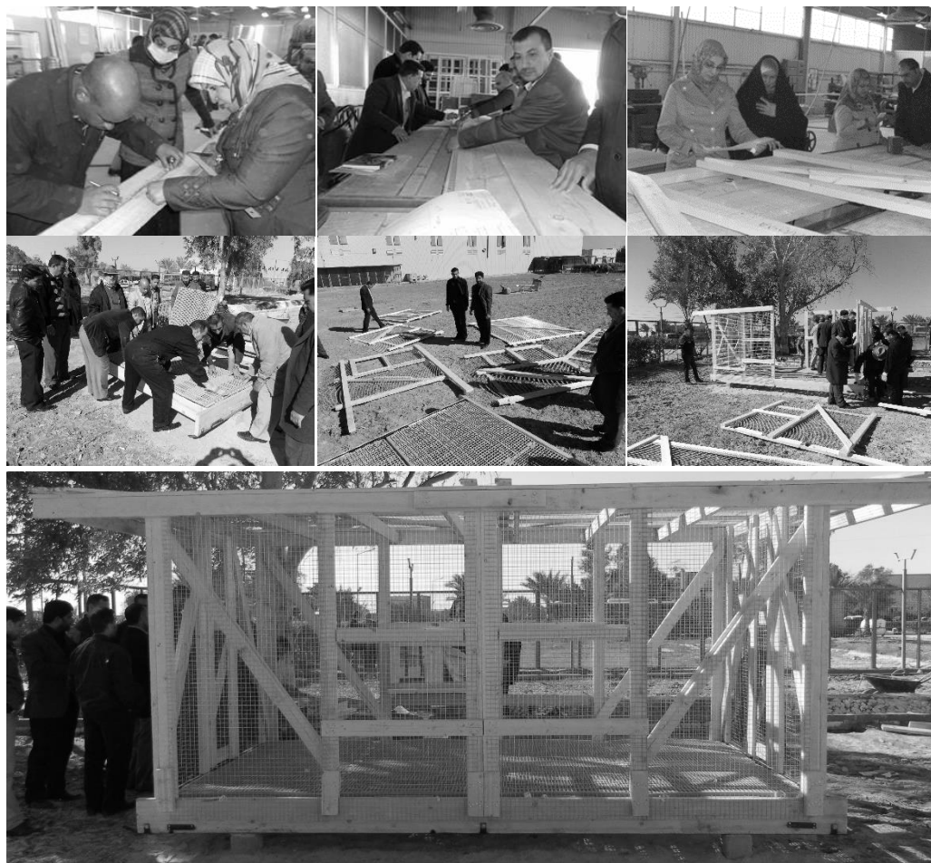
Figure 4. Phases of construction with Iraqi trainees during pilot intervention in the project: ‘Rational management of water resources for agricultural development of rural areas in South Iraq’.
