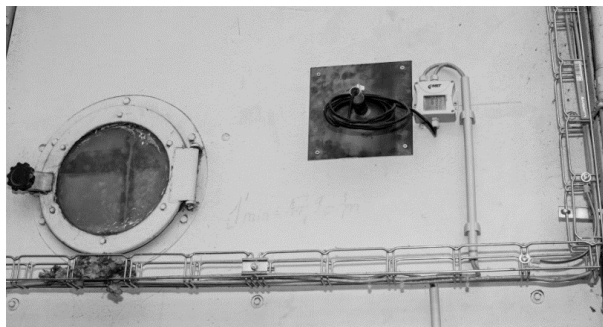
Figure 3. A sensor with transmitter and display installed nearby the dryer check window.
