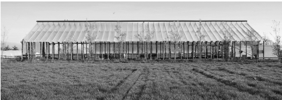
Figure 1. External view of the prototype building used for test.
