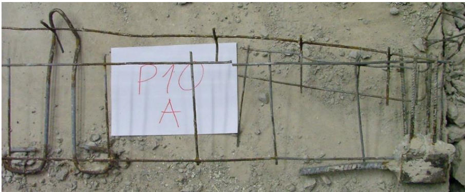
Figure 7. Photograph of the steel prestressing bar, reinforcements and eye bolt details of the longitudinal rib A-B of ribbed panel P10 (P10/A-B) after demolition.
