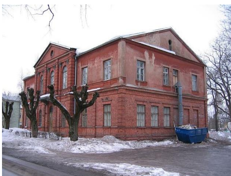
Figure 1. Veski 13 before renovation.
