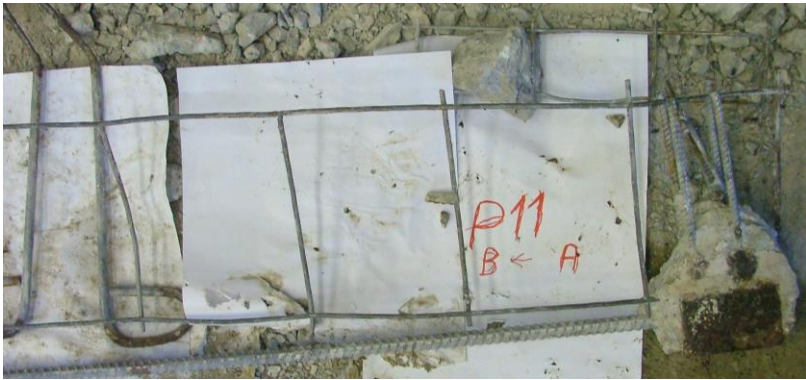
Figure 9. Photograph of the steel prestressing bar, reinforcements and eye bolt details of the longitudinal rib A-B of ribbed panel P11 (P11/A-B) after demolition.
