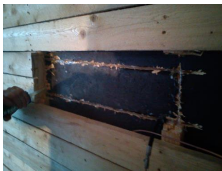
Figure 4. Sealing the opening with silicone.
