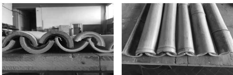
Figure 2. Technique construction of bamboo roofs.
