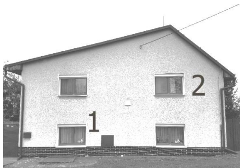
Figure 1. Family house from the north, measured walls are marked.
