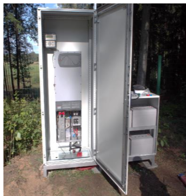
Figure 2. Inverter and batteries in their compartments.
