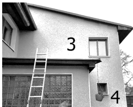
Figure 2. Family house from the south, measured walls are marked.
