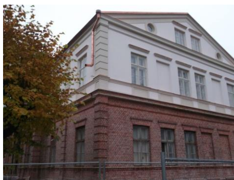
Figure 2. Veski 13 after renovation.
