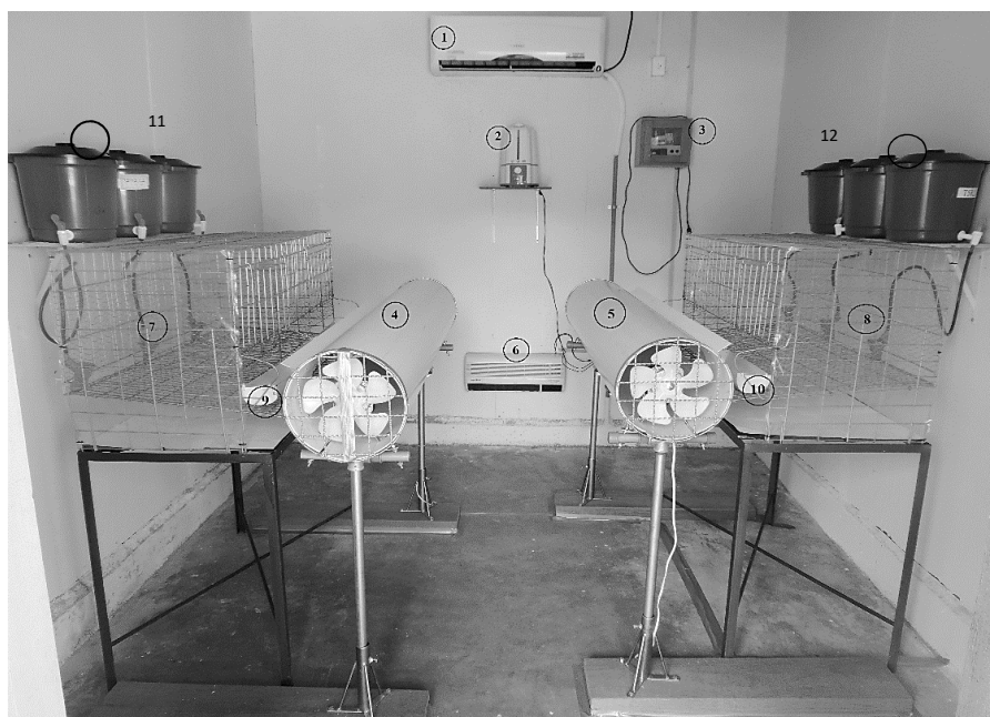
Figure 1. Inside view of the climatic chambers, where 1: air conditioning; 2: air humidifier; 3: electronic temperature and relative humidity controller (MT-531R plus); 4 and 5: ventilation tubes; 6: air heater; 7 and 8: cages; 9 and 10: feeders; 11 and 12: water tanks.
