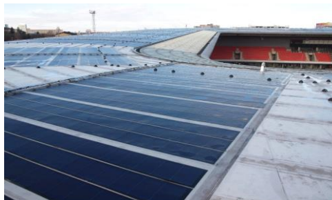
Figure 4. PV system in Prague (Czech Republic) with standard construction with PV panels laid horizontally without supporting stands.
