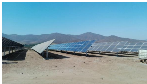
Figure 2. PV system in Cuz Cuz (Chile), advanced construction with tracking stands of PV panels with horizontal tracking axis.
