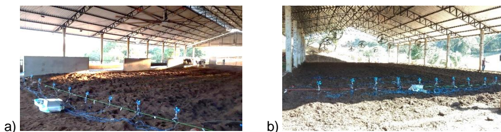
Figure 4. Distribution of the anemometer network in the cattle dairy buildings with compost barn: a) High-volume low-speed fans; b) Low-volume high-speed fans.
