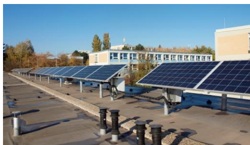
Figure 3. PV system in Prague (Czech Republic) with standard construction with fixed stand of PV panels inclined to the south at an angle of 35^{\circ} .
