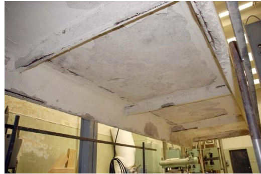
Figure 4. The condition of ribbed panel P8 before testing. Due to corrosion-affected spalled cover at the longitudinal ribs, ribbed panel P8 received grade 0 in the visual rating scale.
