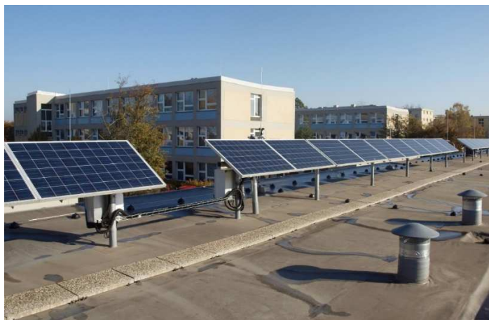
Figure 1. On-grid PV system installed at the Faculty of Engineering, Czech University of Life Sciences Prague (nominal output power 10 kW_p ).
