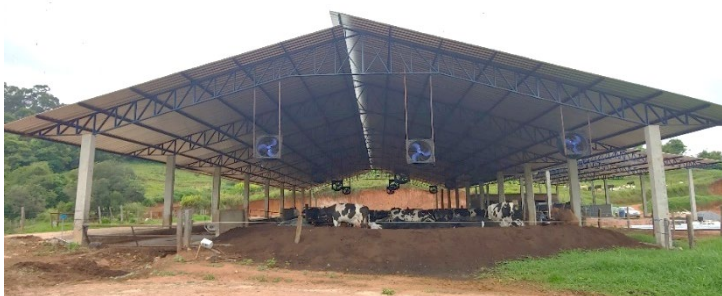
Figure 2. West side view of the Compost Barn.
