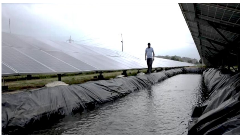
Figure 6. Fish Pond set-up underneath PV-modules in Bhaloji, Rajasthan, India (National Solar Energy Federation of India. 2023).
