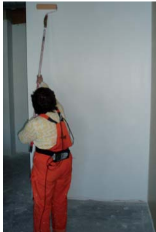
Fig. 1. Performing a 3-minute wall painting test.
