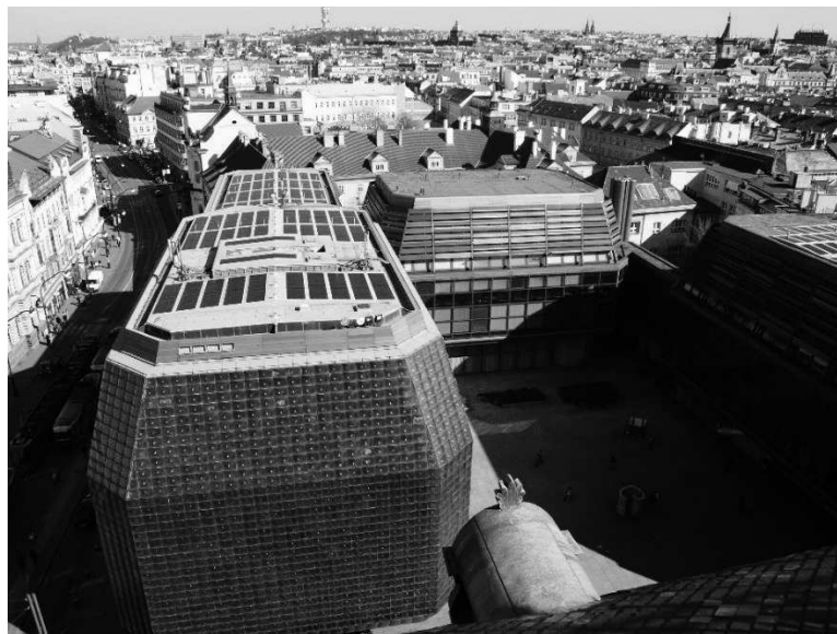
Figure 1. PV power plant on the National Theatre roofs (New Scene Building left, Service Building right).
