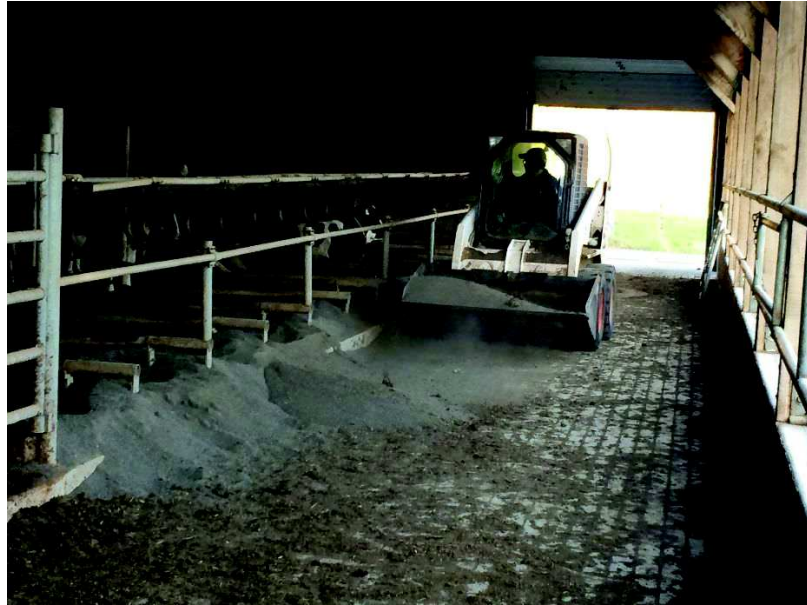
Figure 2. Lost sand in the connecting alley – part of the investigated barn.
