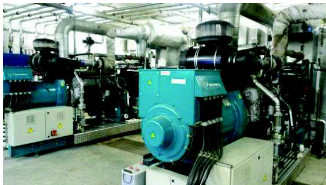
Figure 2. Cogeneration units.
