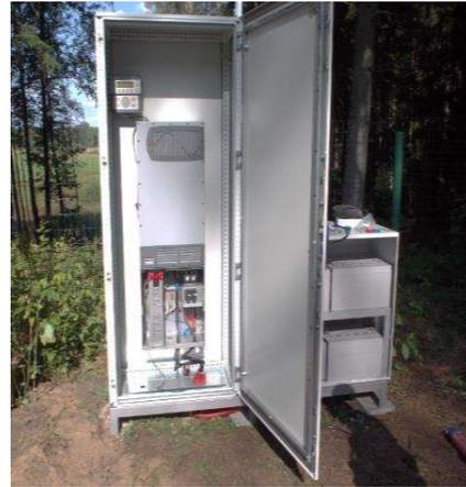
**Figure 2.** Inverter and batteries in their compartments.
