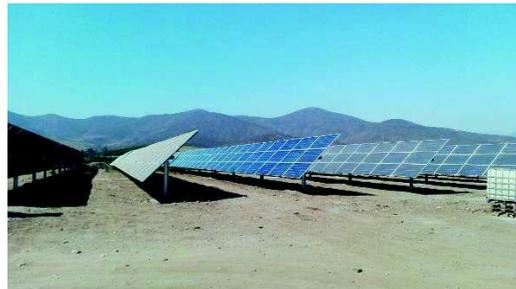
**Figure 2.** PV system in Cuz Cuz (Chile), advanced construction with tracking stands of PV panels with horizontal tracking axis.
