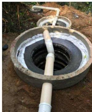
**Figure 4.** Tanks prepared to receive the lid.
