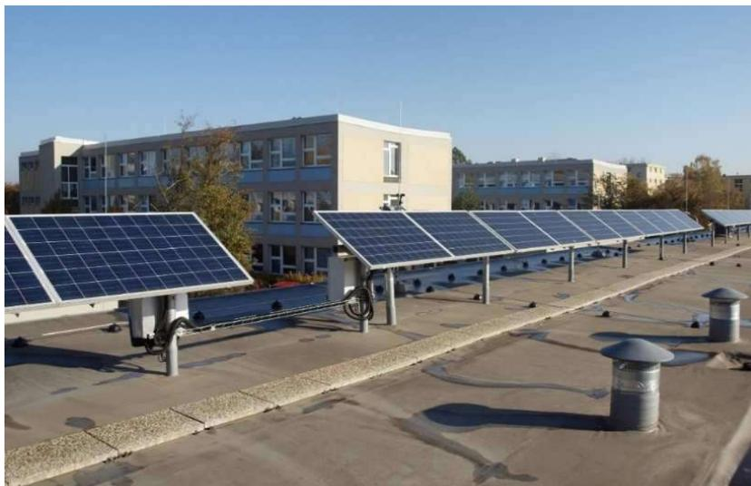
**Figure 1.** On-grid PV system installed at the Faculty of Engineering, Czech University of Life Sciences Prague (nominal output power  $10 kW_p$ ).
