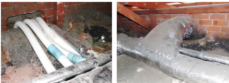
Figure 2. Air ducts coming from the facade into the attic (without insulation and already insulated).
