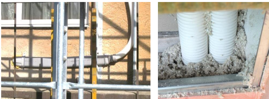
Figure 1. Air ducts are mounted into the facade's insulation layer, enter the living room through the wall directly behind the heating radiators.
