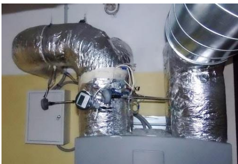
Figure 3. Placement of the combined airflow and temperature transmitter.
