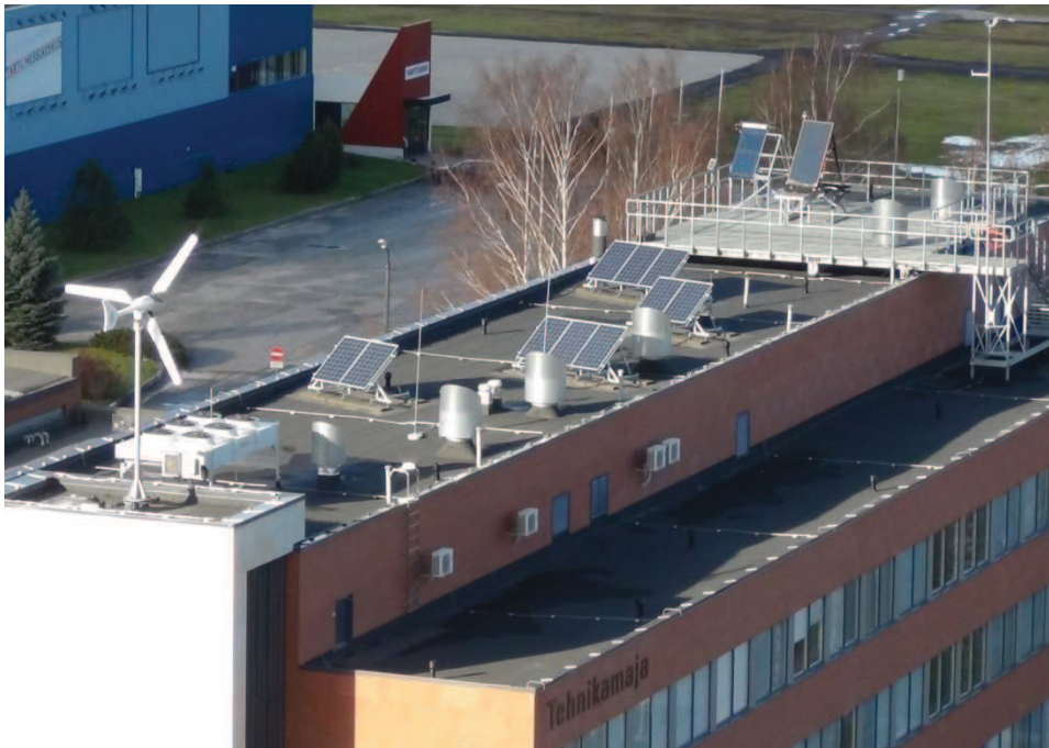
Figure 5. Equipment on rooftop.
