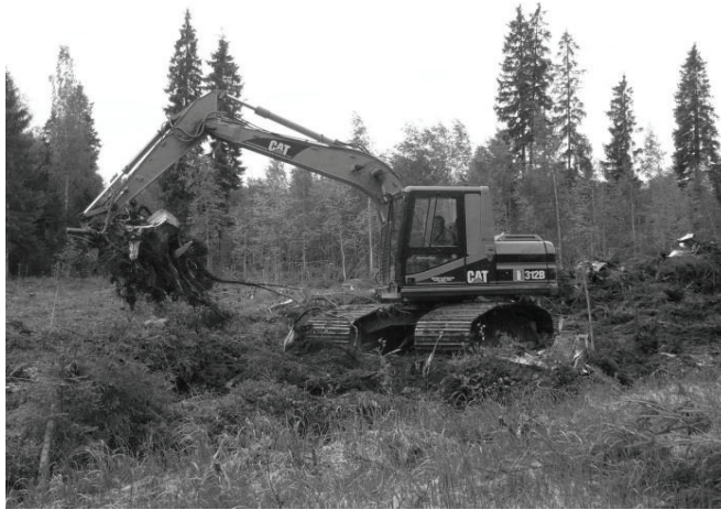
Figure 1. Excavator in stump-root system extraction on one peatland forest site (Jussi Laurila).
