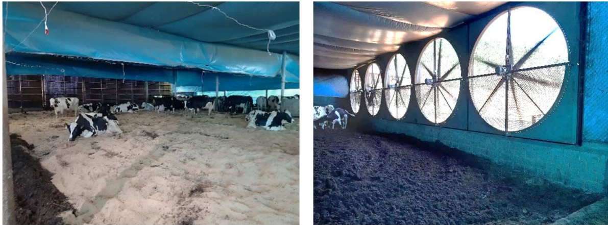
Figure 1. The compost barn with tunnel ventilation: deflectors (left) and large fans (right) are shown.
